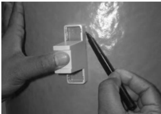
Hold the tank sensor plastic housing against the insulation and mark an outline.
